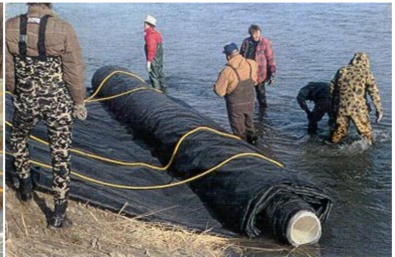
2. Ropes extend to circle under AquaDam® and back to anchor pipe. On bank the AquaDam® begins filling.
