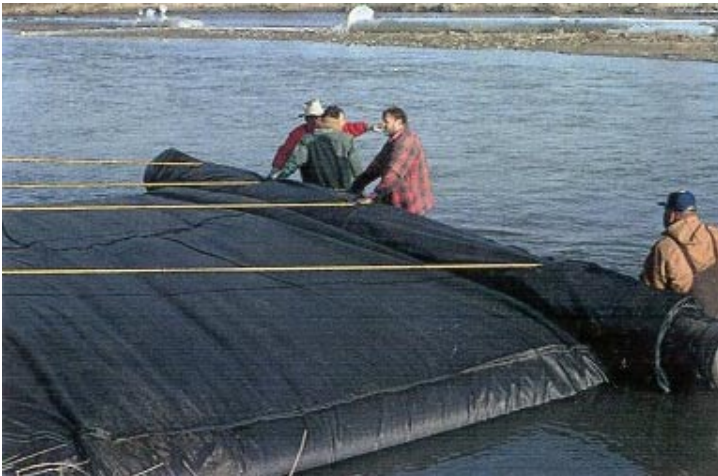
3. Ropes keep the AquaDam® from unrolling. Water head builds inside.
