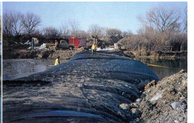
6. This AquaDam® is big! Made with over 70,000 gallons of water!
